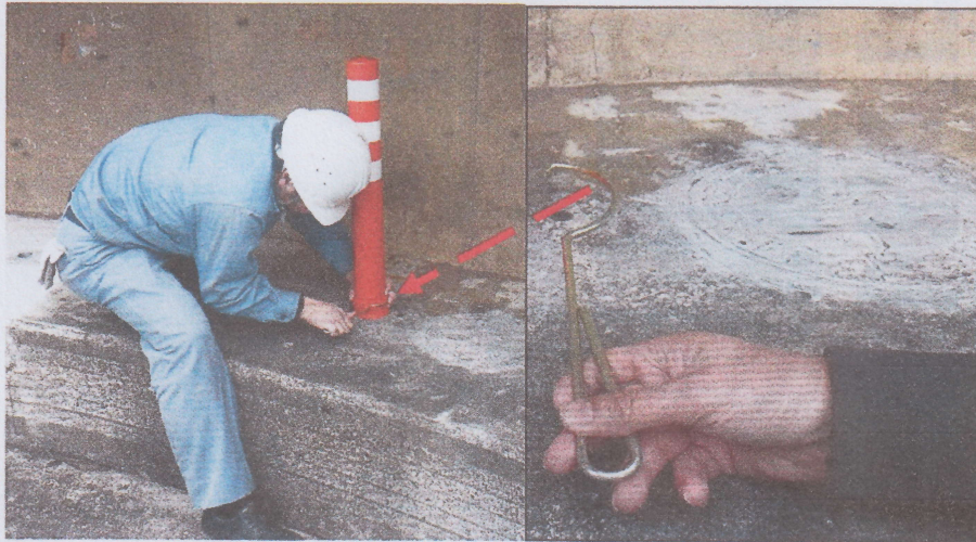
Photo 1: Pole cone must be fastened completely with the torque 106 N.m using special installation tool (SJC tool)
